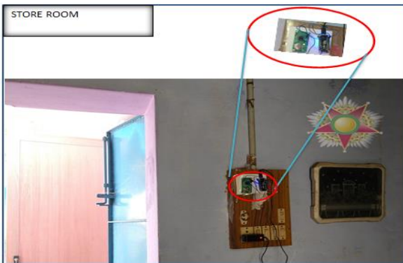
Figure.2 c Sensor 'S1' fixed at Store Room
